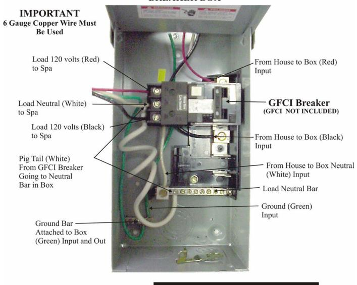
NOTE: The White Neutral Wire from the GFCI MUST be connected to an incoming Line Neutral. The internal mechanism of the GFCI requires this Neutral connection. The GFCI **WILL NOT** WORK WITHOUT IT.
